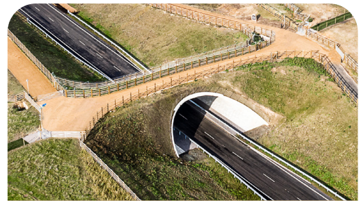
GREEN BRIDGE WITH FOOTPATH
