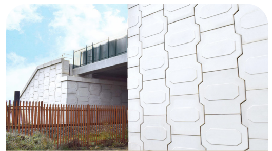
RAIL ABUTMENT BRIDGE
