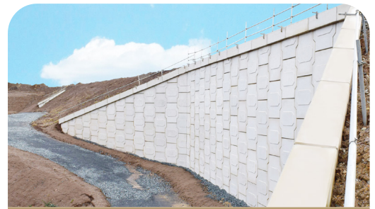
RETAINED EARTH WALL
