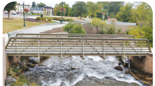
ASSET FRP ACCESS BRIDGE
